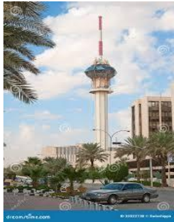
Riyadh TV Tower
